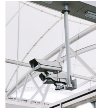
Surveillance Works with IP Cameras
